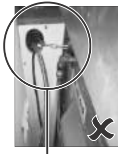
Hole in cabinet too large, allowing the upright oven to tilt forward
