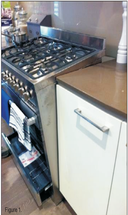
Hole in cabinet too large, Allowing the upright oven to tilt forward
